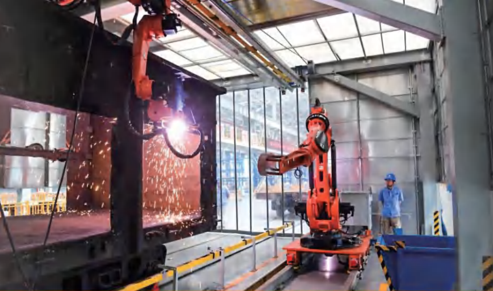
The transfer cart with the mechanical arm makes the working more convenient.
